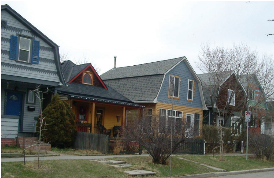
Another variation of the gable-front home in Ramsay is the gambrel roof with dual pitched gable; above is the 1000 block of 18 th Avenue S.E. (Credits: City of Calgary).
