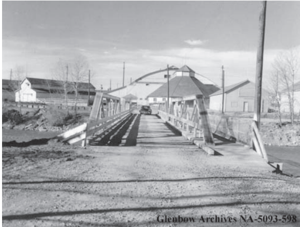
Stampede Park Truss Bridge (installed some time before 1955 and possibly moved from another location) vehicular steel bridge with wood deck in 1958 and 2012. (Credits: Glenbow Archives na-5093-598, R.K. Williams)
